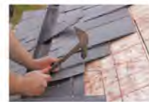
△ Fig. 1.6 Slate being used for roofing.
